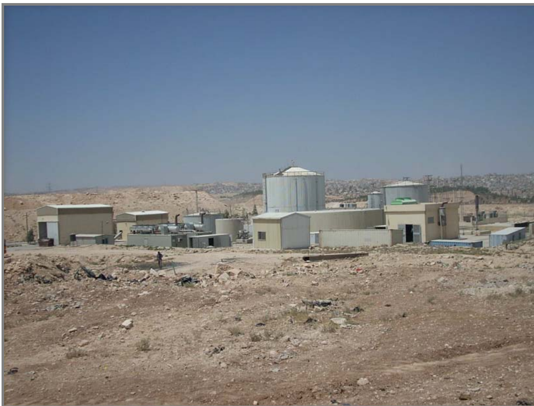
Figure 1 The Ruseifah Biogas Plant with in the centre the biodigester.
